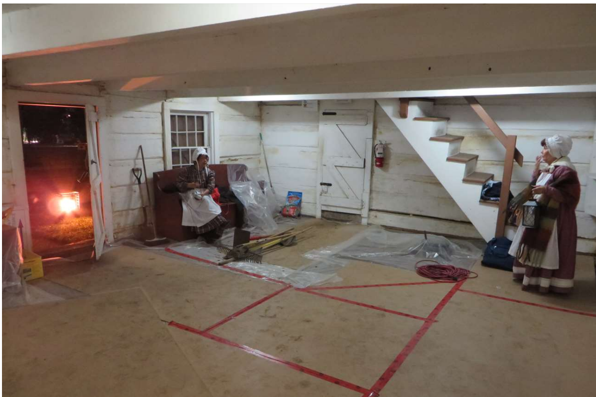
Above: Volunteers Diane Reid and Kayoko Smith admire the repairs in an empty Scadding Cabin while preparing for the Ghost Walk. Photos: Brent Cunningham
